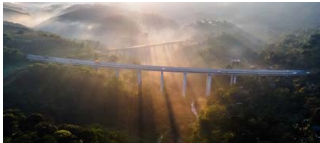
PICTURE FROM GCCA CONCRETE IN LIFE COMPETITION 2023 BY @THE_AMATEUR_PHOTOGRAPH, WEST JAVA," INDONESIA TRANSPORTATION INFRASTRUCTURE IS ONE OF THE IMPORTANT THINGS IN CARRYING OUT THE COUNTRY'S ECONOMIC ACTIVITIES."
