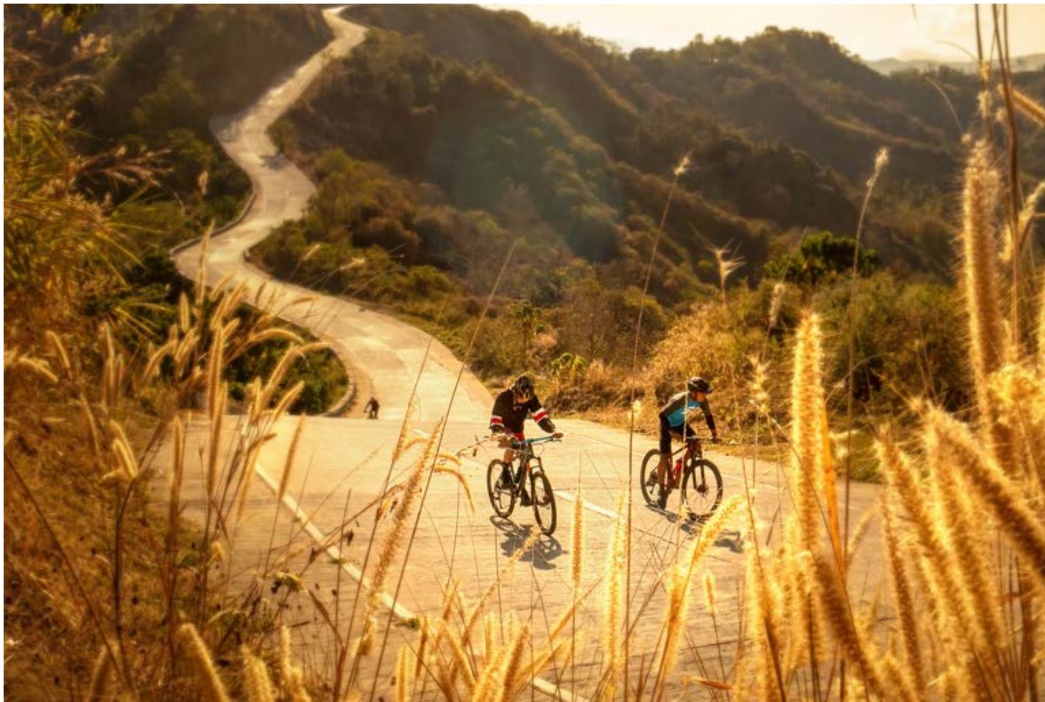
PICTURE FROM GCCA CONCRETE IN LIFE COMPETITION 2023 BY @DANVICPHOTOS LA UNION, PHILIPPINES, "THE NEWLY CONSTRUCTED 10 KILOMETER UPLAND CONCRETE ROAD SIGNIFICANTLY IMPROVED THE ROAD SAFETY AND REDUCE TRAVEL TIME FROM A 5-HOUR HIKE TO A 15 MINUTES DRIVE THIS IS THE ROUTE GOING TO SASABA RICETERRACES AND SIMMINUBLAN FALLS IN LA UNION, PHILIPPINES"
